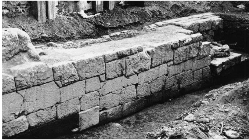
Figure 22. Themistoklean course, stretch of curtain wall at Erechtheiou 20 (Th86); view from the southwest. Lowest course of reused material; second through fourth courses of limestone blocks, smaller in second and third courses, built in polygonal masonry tending toward trapezoidal; all-stone construction on preexisting foundations (at rear). Travlos, Attika , p. 174, fig. 226. Photo © Ernst Wasmuth Verlag GmbH & Co.
