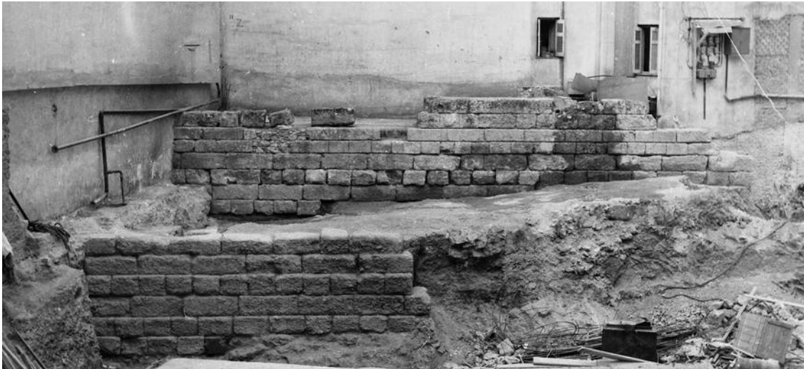
Figure 31. All-stone Hellenistic construction at the intersection of Aristeidou 14 and Pasmazoglou Street (Th29). Curtain wall at rear. External ring road (middle); pro-teichisma (foreground). Travlos Archive, photography folder 112 (Photographs from Athens). Courtesy Archaeological Society at Athens
