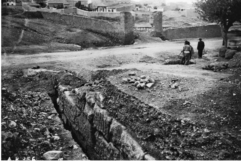
Figure 27. Themistoklean course, stretch of curtain wall in front of Erysichthonos 17 (Th106); view from the northeast. Irakleidon Street at rear. Photo courtesy Deutsches Archäologisches Institut (neg. D-DAI-ATH-Athen Bauten 356)
