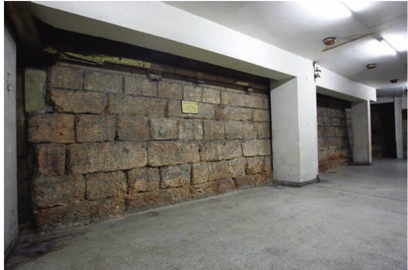
Figure 36. Hellenistic curtain wall of all-stone construction at Dragatsaniou 6 (Th32). Photo A. M. Theocharaki
