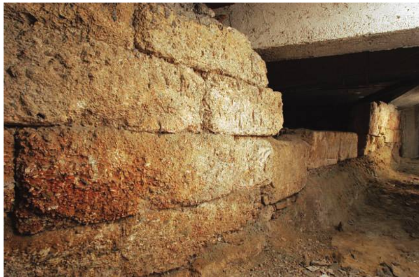
Figure 33. Themistoklean course, southern curtain wall at Dipylou 5–7–9 (Th9); view from the southwest. Reused poros block (center); limestone blocks on poros stretchers (at rear); conglomerate stretchers (foreground). Photo A. M. Thecharaki
