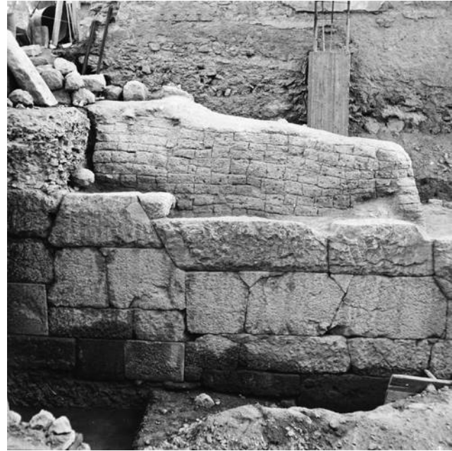
Figure 23 ( left ). Fill between the two stone faces of curtain wall, Erysichthonos 15 (Th109). Photo G. Hellner, courtesy Deutsches Archäologisches Institut (neg. D-DAI-ATH-Athen Bauten 673)
