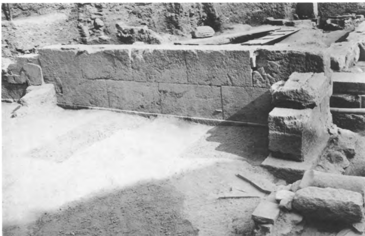
a. Detail of south wall of south room, from northwest, showing original doorway
