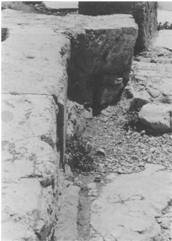
a. Eastern end of Bedding A, southern edge, from west
