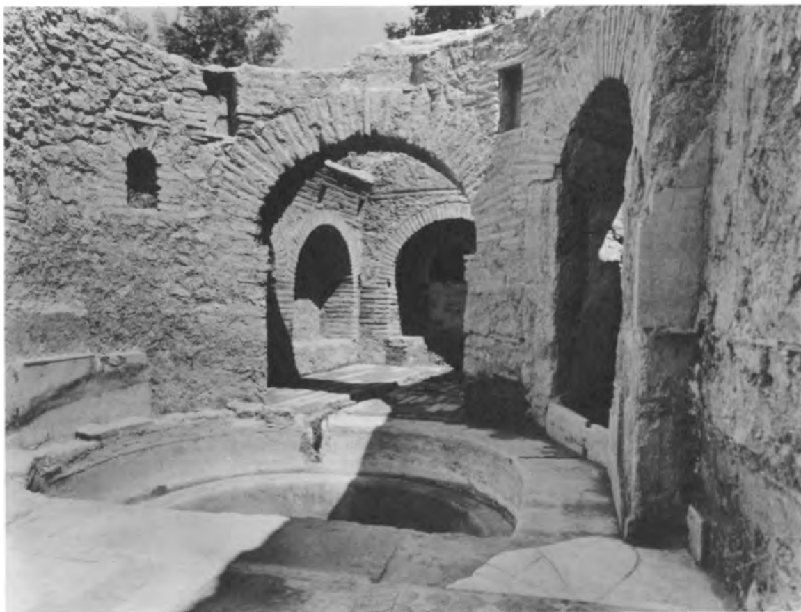
a. Apsidal Suite from Southwest, showing Pool and Inner Vaulted Chamber
