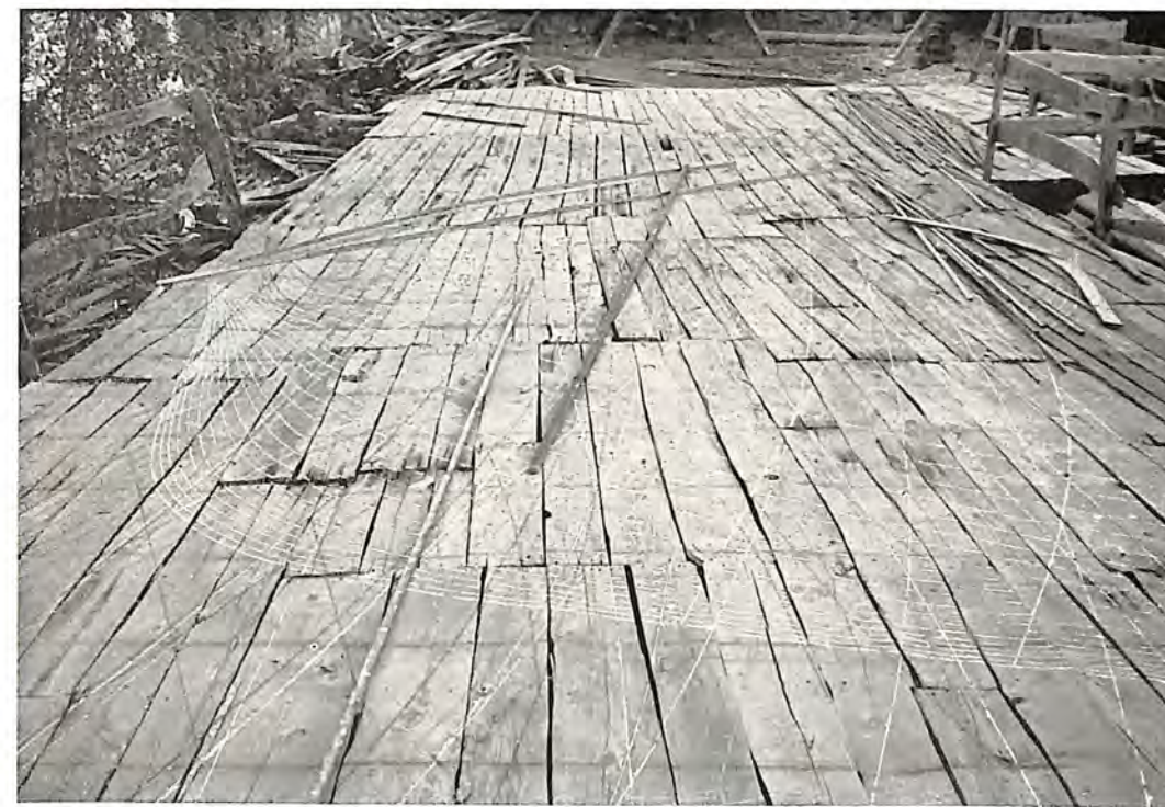
Figure 12. Moulds laid out on a scribe board, at George Mavrikos' yard in Syros. Battens make it possible for the designer to obtain fair lines to 1:1 scale, which then can be transferred to shapes of frames. This invention made the use of tenons unnecessary.
