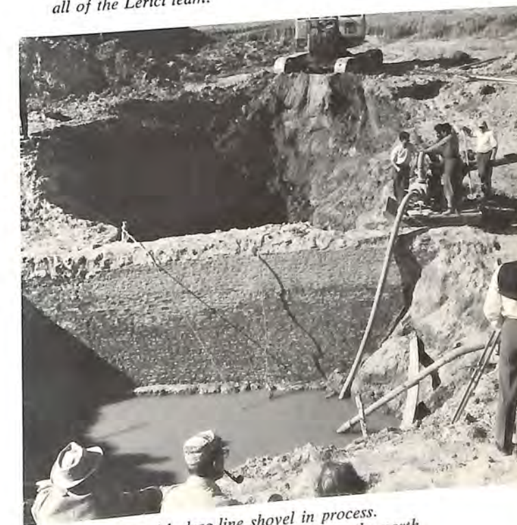
Jeep-mounted drill with forced water circulation. The cuttings are being scooped up with a shovel. At right are Franco Brancaloni and Marjolein deVos and at left (wearing straw hat) is Giuseppe Cesari, all of the Lerici team.
