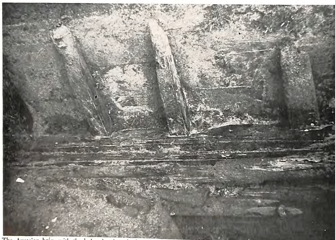
The Austrian brig, with the bulwarks cleared of mud. Note that the lower parts of the timbers still shine with their original oiled finish. The upper parts of the timbers and the cap rail have been eaten by teredo worms.
