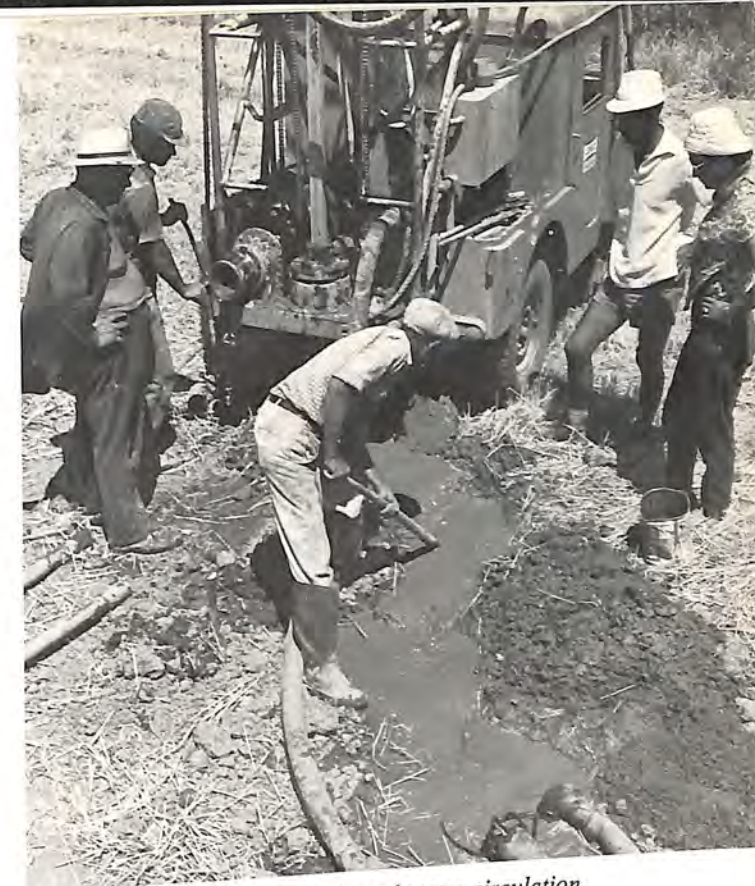
Jeep-mounted drill with forced water circulation. The cuttings are being scooped up with a shovel. At right are Franco Brancaloni and Marjolein deVos and at left (wearing straw hat) is Giuseppe Cesari, all of the Lerici team.
