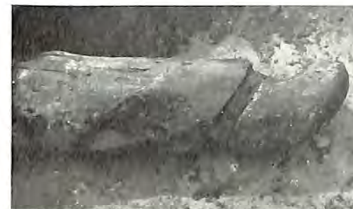
Figure 22. Beam GXM after removal. Slot in side fits filler planks. See Fig. 20.
