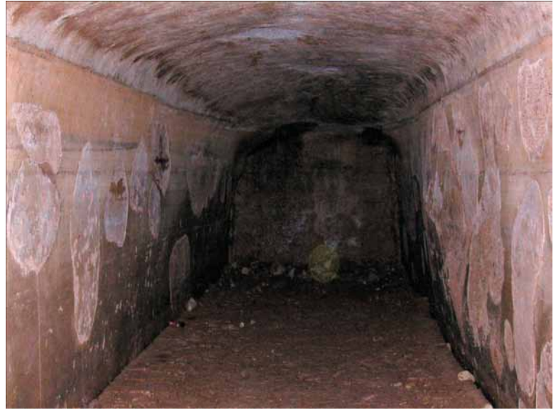
Figure 10. Peirene: View south into Reservoir 3, showing hydraulic mortar and lime encrustation
