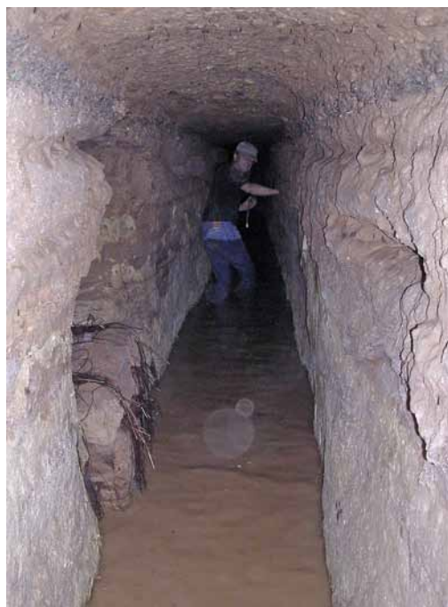
Figure 18 (left). Peirene: View north in south-central supply tunnel under the forum, with Paul Scotton for scale. Visible on the left is the unexplored channel between Manholes H and J.
