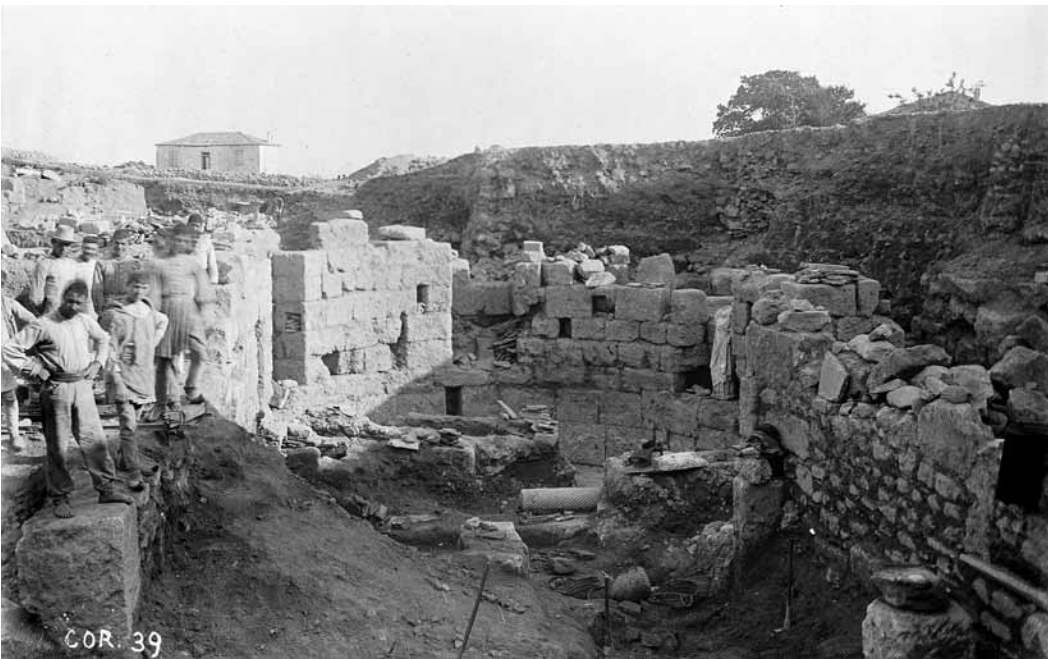
Figure 45. Peirene: North apse on or about May 30, 1898, with Early Byzantine tombs just right and left of center, and later medieval walls to right and left
