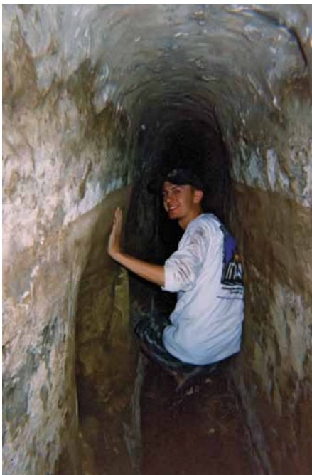
Figure 14. Peirene: Forward cross-tunnel, view east showing funnel-shaped opening into a reservoir, with Eric Maxeiner for scale
