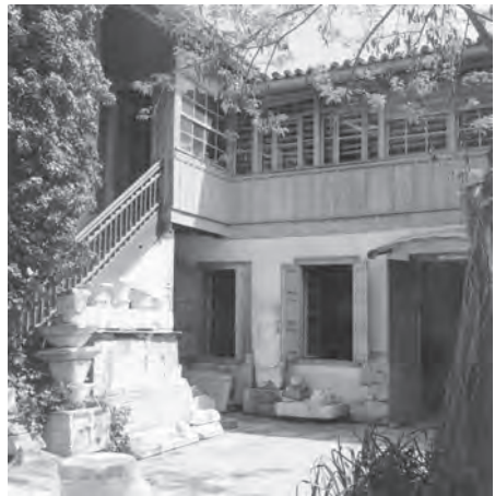
Figure 2. Courtyard of the old excavation house
