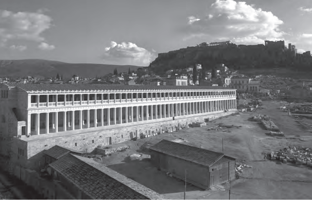
Figure 3. The Stoa of Attalos after reconstruction (1956)
